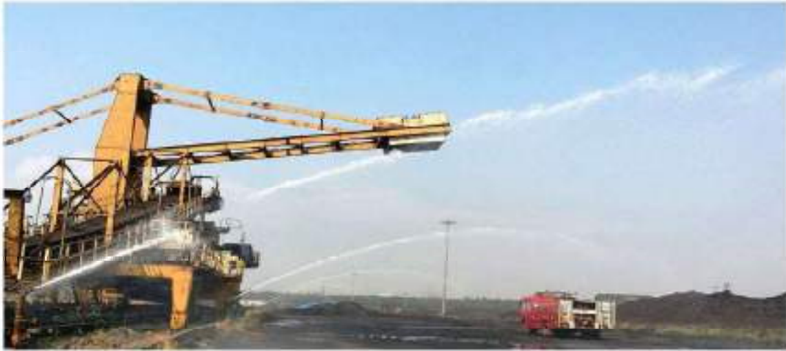
WATER SPRINKLERS AT COAL STACK YARD
