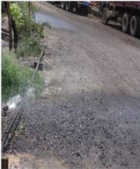
WATER SPRINKLER AT COKE OVEN AREA
